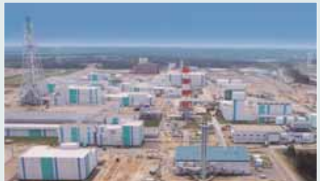
Nuclear fuel reprocessing facility
