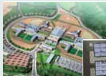
Overview of the finished installation
