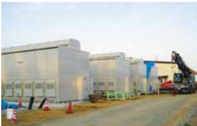
Battery storage system for wind power generation plant
