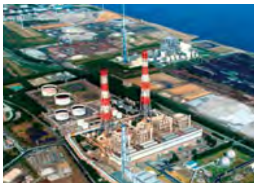
Kashima Kyodo Electric Power's generation facility
