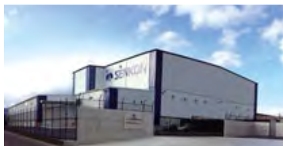
New Fukushima warehouse
