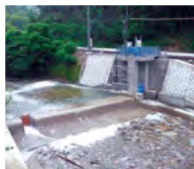
Funama power plant, under construction
