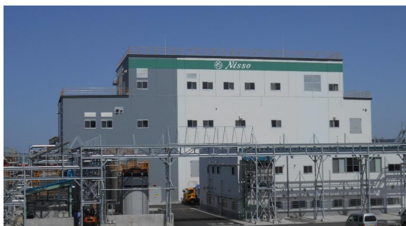
Nihongi Plant Expanded production facility of Pharmaceutical additive NISSO HPC
