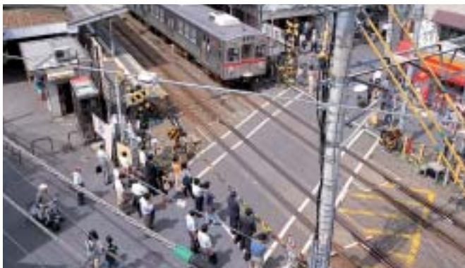
Before elevated crossing
