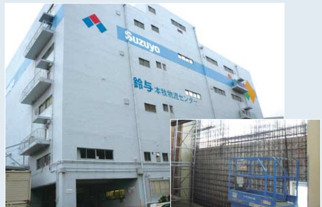
Earthquake reinforcement construction is underway at a Suzuyo shipping facility
