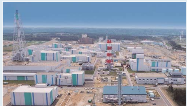
The Rokkasho Nuclear Fuel Reprocessing Facility
