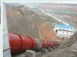
Hydro Power Project Kanfeng in China
