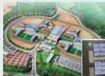
Overview of the finished installation
