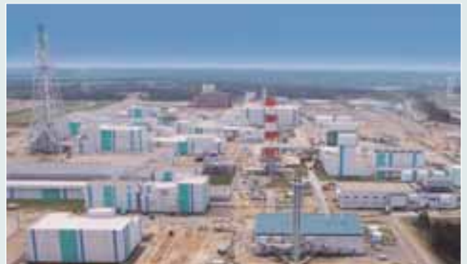
Nuclear fuel reprocessing facility
