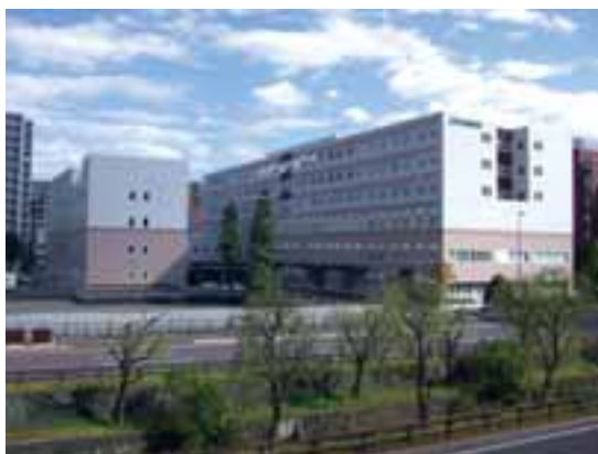
JR Sapporo Hospital after reconstruction
