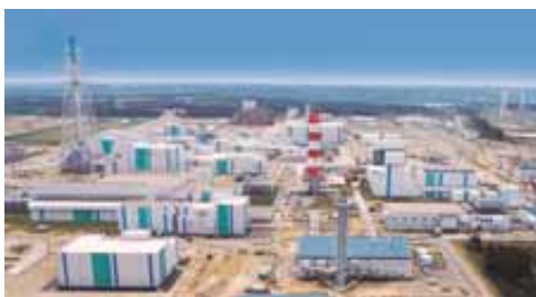
Nuclear fuel reprocessing facility
