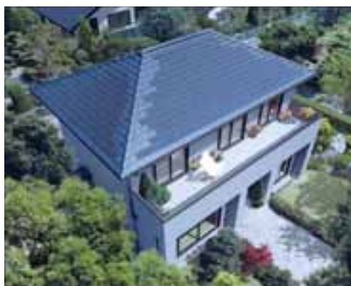
Hybrid photovoltaic cell (thin-film photovoltaic cell) used on home rooftop
