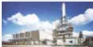
Nakayama Joint Power Generation Co., Ltd.: Independent power producer (IPP) power generation operations (Osaka Prefecture) In step with relaxation of regulations, project finance support for Japan's first steelmaker to enter the power generation business
