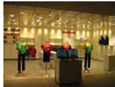
Showroom for proposing and displaying energy-efficient lighting solutions
