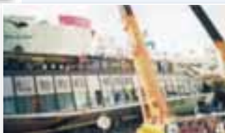
Hankyu Corporation: Earthquake reconstruction work (Hyogo Prefecture) Recovery work on traffic infrastructure destroyed by earthquakes
