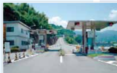
Toyo Tires Turnpike (formerly the Hakone Turnpike) DBJ established Japan's first infrastructure fund in collaboration with Australian investment bank Macquarie Bank, involving equity investment to facilitate business transfer transactions for the former Hakone Turnpike.
