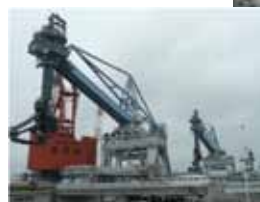
Coal unloader repaired after the earthquake
