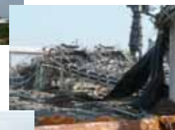
Coal unloader after the earthquake
