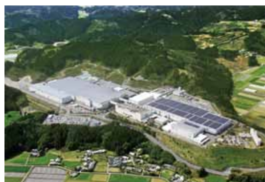
Solar Frontier's Kunitomi Plant
