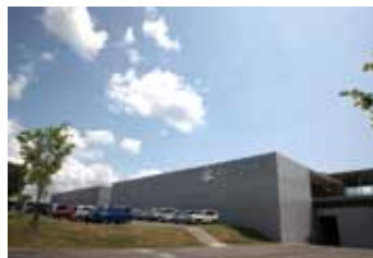
Headquarters and factory exterior
