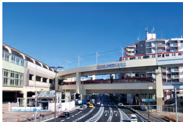
Continuous grade separation project
