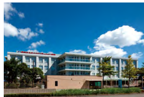
Yokohama Namiki Rehabilitation Hospital
