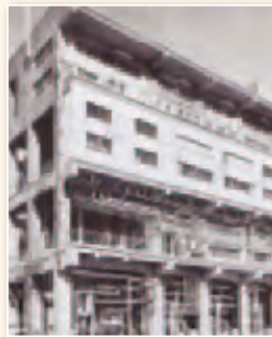
Asahi Chemical Industry Co., Ltd. (currently Asahi Kasei Corporation): Construction of the Fuji Plant for production of Cashmilon acrylic staple fiber (Shizuoka Prefecture)
