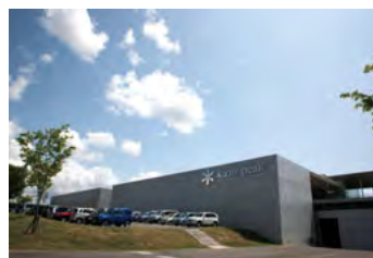
Headquarters and factory exterior
