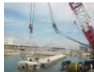
Quay wall construction
