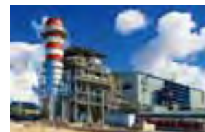
EPEC's gas-fired thermal power generation facility
