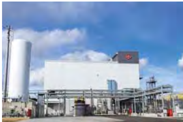
External view of new annex at Sukagawa Plant
