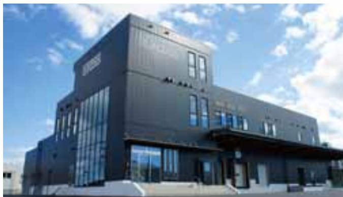
External view of head office factory
