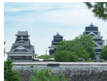
Kumamoto Castle, damaged by the earthquakes (photo from the Ninomaru Parking Lot)
