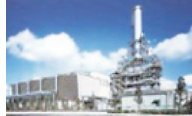
Nakayama Joint Power Generation Co., Ltd.: Independent power producer (Osaka) JDB offered project finance for Japan's first steelmaker to enter the power generation business triggered by deregulation.
