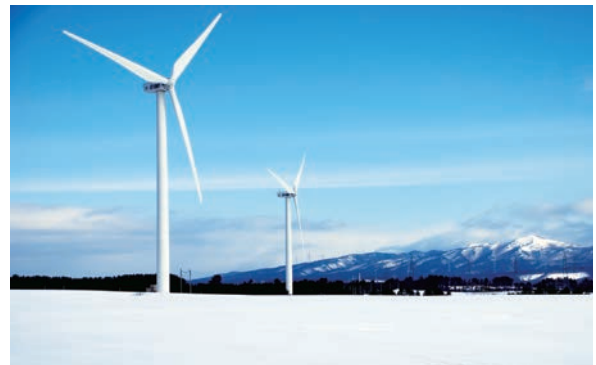
Japan Wind Development Co., Ltd. facilities
