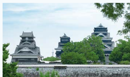
Kumamoto Castle, damaged by the earthquakes (photo from the Ninomaru Parking Lot)
