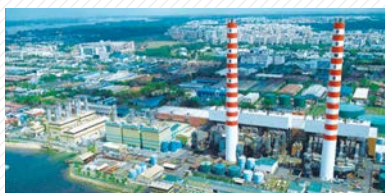
Senoko Power Ltd. (Singapore) DBJ provided subordinated financing to Senoko Power, the largest electric power company in Singapore.
