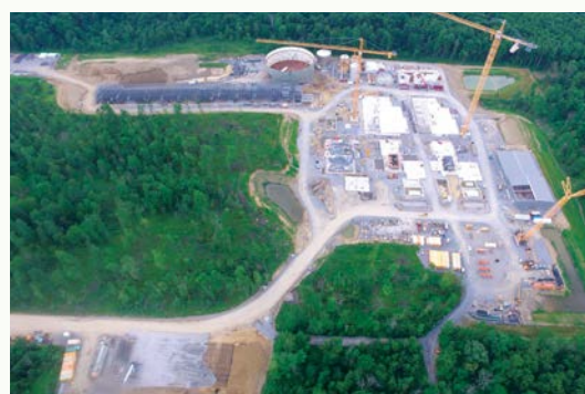
Power plant under construction
