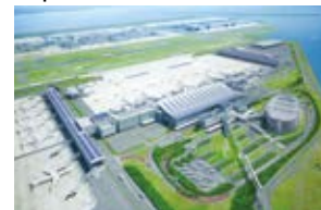
Tokyo International Air Terminal Corporation
