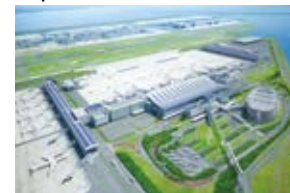
Tokyo International Air Terminal Corporation
