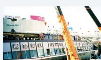
Hankyu Corporation: Earthquake reconstruction work (Hyogo Prefecture) Recovery work on traffic infrastructure destroyed by earthquakes
