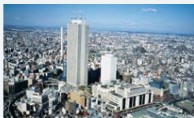
New Town Center Development Co., Ltd. (Now Sunshine City Corporation): Sunshine City construction (Central Tokyo) Ikebukuro redevelopment for new urban configuration
