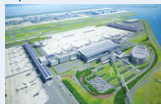
Tokyo International Air Terminal Corporation
