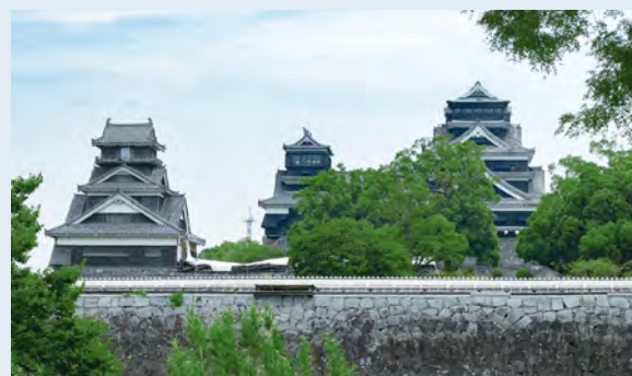
Kumamoto Castle, damaged by the earthquakes (photo from the Ninomaru Parking Lot)
