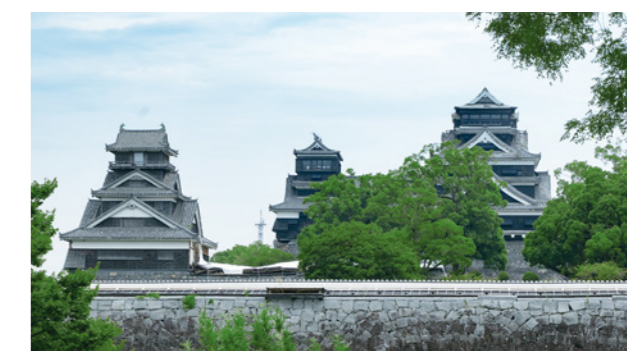
Kumamoto Castle, damaged by the earthquakes (photo from the Ninomaru Parking Lot)
