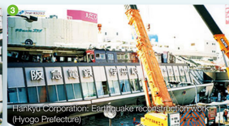
Recovery work on traffic infrastructure damaged by the earthquake
