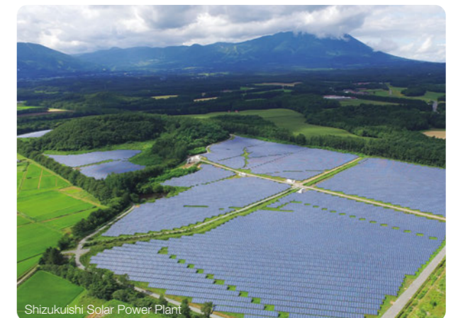
Shizukuishi Solar Power Plant
