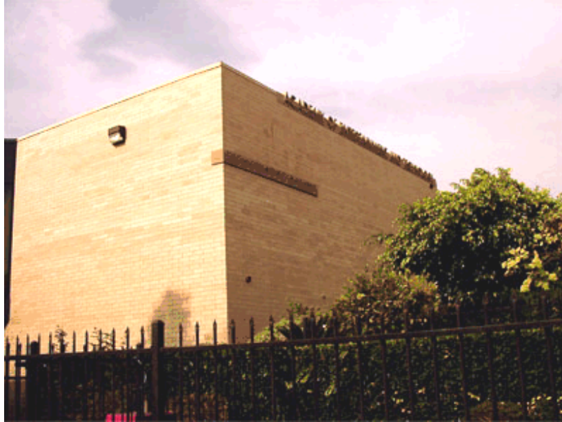
Academy of Entertainment & Technology Building
