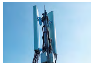
Cellnex Telecom, S.A.
