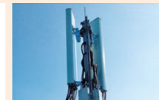
Cellnex Telecom, S.A.
